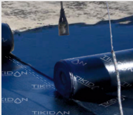
TORCHING AND LAYING OF MEMBRANE
