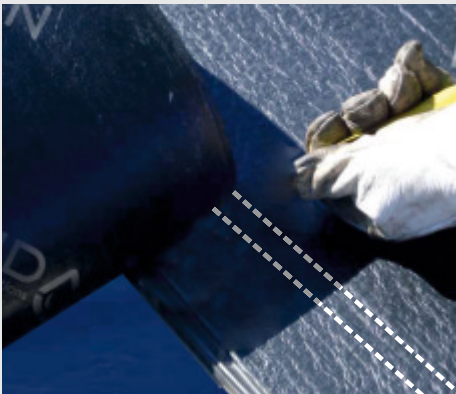
MAINTAIN OVERLAPS AS PER MARKINGS
