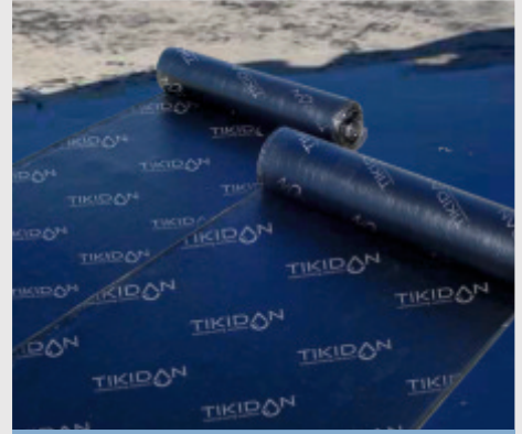
ALIGNMENT & REALIGNMENT OF MEMBRANE ROLLS
