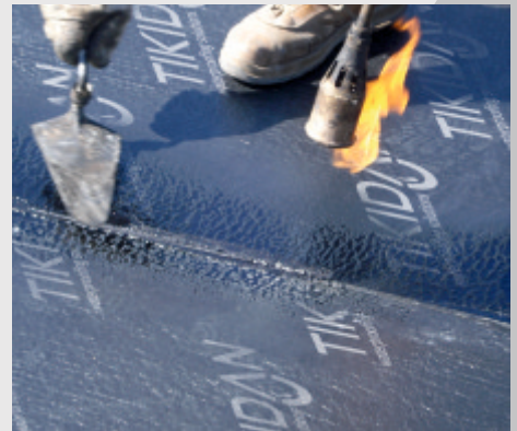
WATERTIGHT SEALING OF SEAMS
